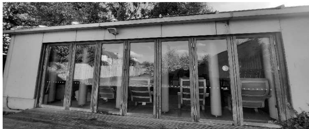
Back façade—sliding wood and glass doors that provide ventilation and lighting
