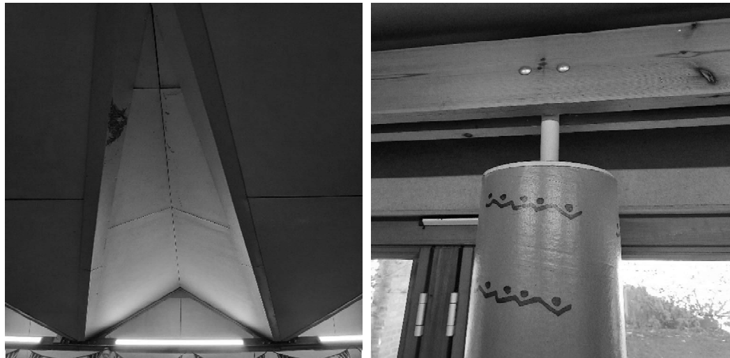
Connection between paper tube column and wood truss
