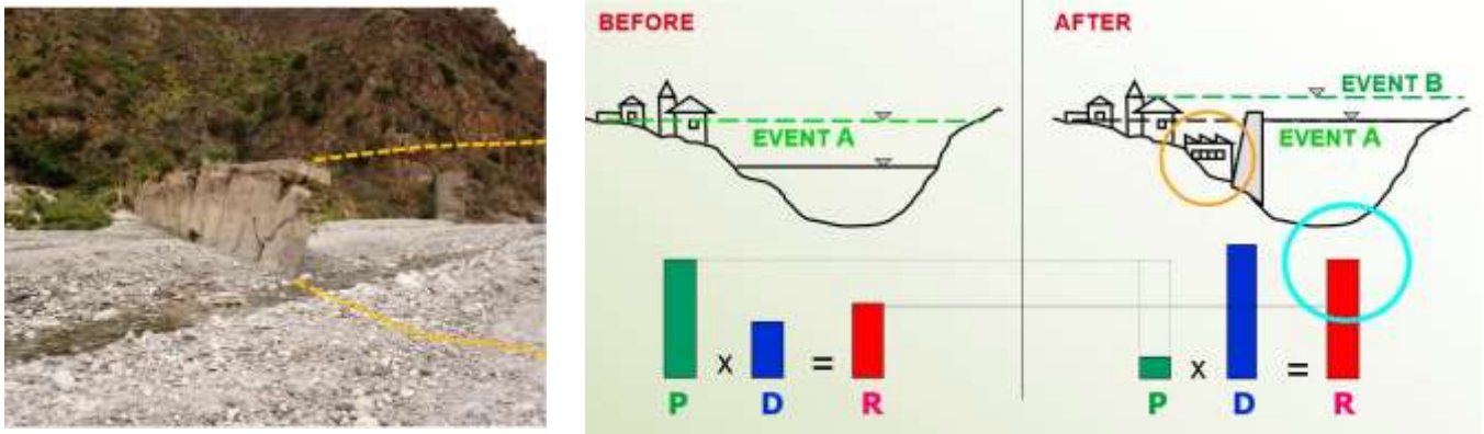
Figure 2. (Left): Evidence of two failed big weirs originally conceived to control downstream aggradation: a stout, but fragile, solution; (Right): The paradox of putting a system in safe conditions leading to an increase in risk with respect to the original situation (BEFORE sketch) because people, feeling safe after the protection works (the longitudinal dike in the AFTER sketch), inevitably increase exposed value (golden circle and higher blue D bar of potential damage; not in scale); but an event higher than the design one (Event B higher than Event A) is perfectly possible, although with a lower occurrence probability (P); Risk (R), a combination of probability P and damage D, has hence grown.
