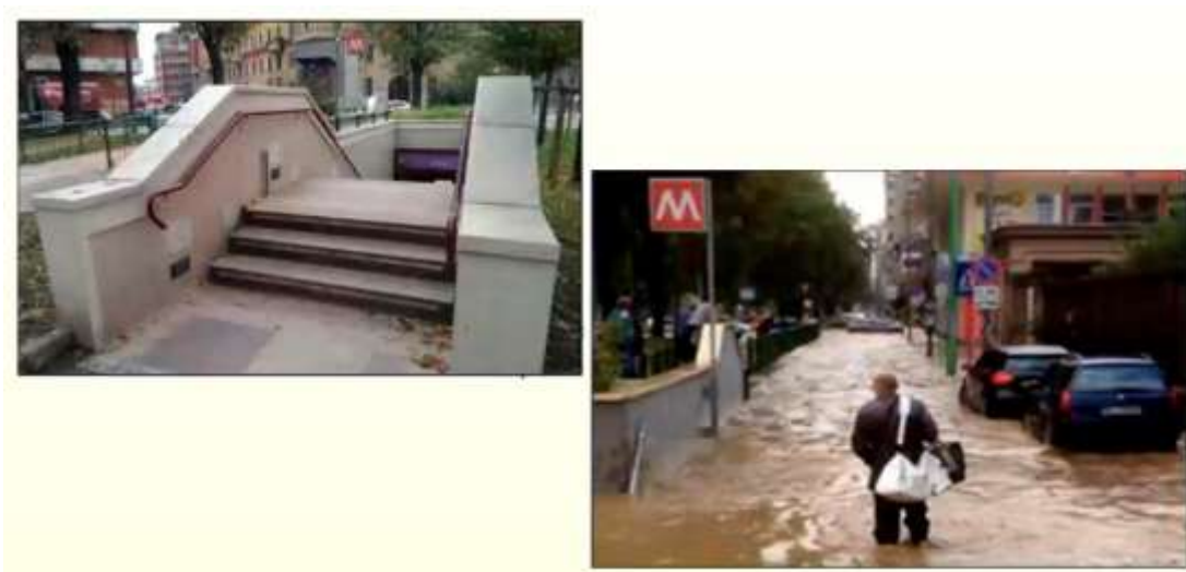
Figure 8. Example of water proofing intervention: (left) raised elevation of the contour of the access facility to a Metro MM5 station in Milan; (right) the same access proving to impede water entrance into the station, while keeping its full functionality, during a harsh flood from Seveso river in 2014 (by kind permission of Daniele Bignami, Politecnico di Milano, FLORIMAP project, Fondazione Cariplo, Milano, I).
